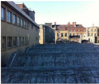
Asphalt Roofs Before
